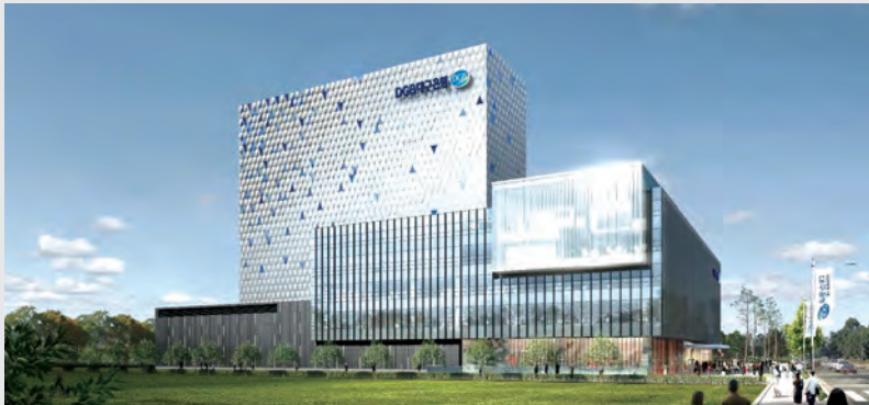
Daegu Bank (DGB) Data Center (PreCon)
