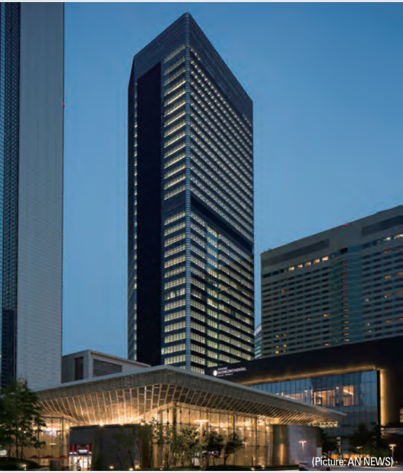
Parnas Tower (PreCon)
